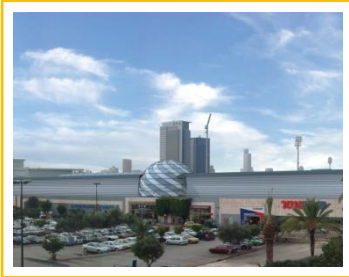
Azrieli Ayalon mall (additional floor) Approx. 9,500
